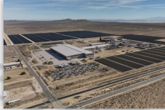
PSG MOJAVE STEEL MILL (CEC) 32 MWh Endurium / California
