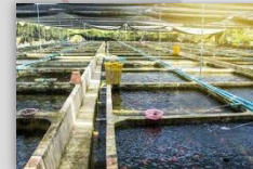
CHARLES MURGAT 3.5 MWh / Lyon
