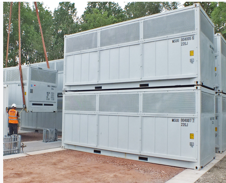
Siting underway. Double-stacked configuration shown
