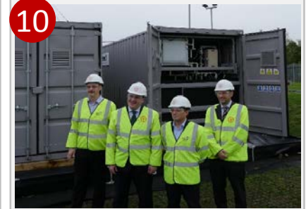
10 Large Machines tested with SSE at PNDC site
