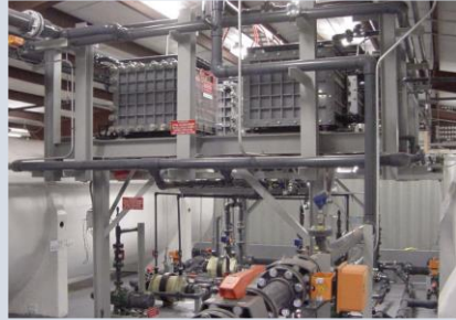
VRB Power delivers 2 MWh flow battery to Pacificorp, Utah, USA
